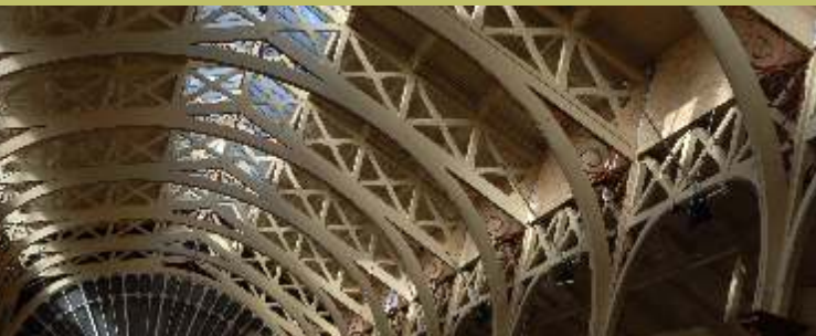
The architectural roof of Barnstaple's historic market
